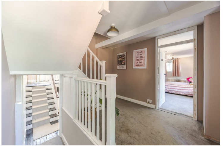
Landing 2nd floor
